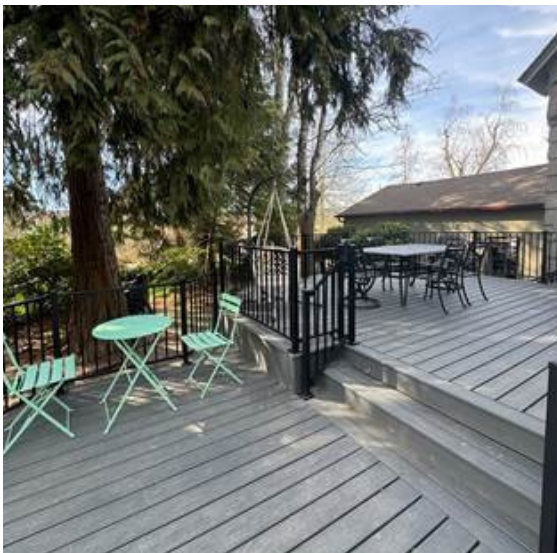
New deck at David's House. Photo credit: MWVCAA
